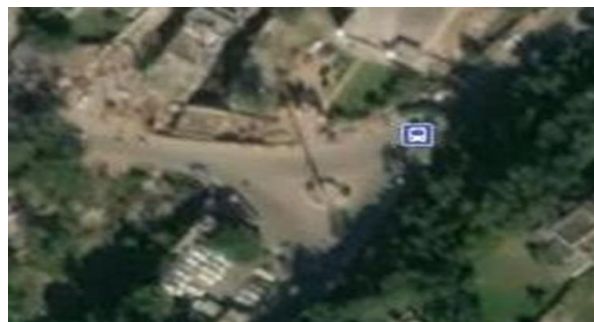
Fig 2 : shows intersection of road Source: google earth
